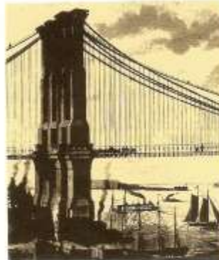
Suspending the floor beams, 1880.
